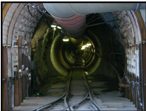
Innergex Ashlu Project Tunnel
