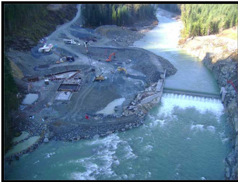
Ashlu Creek Intake and Weir
